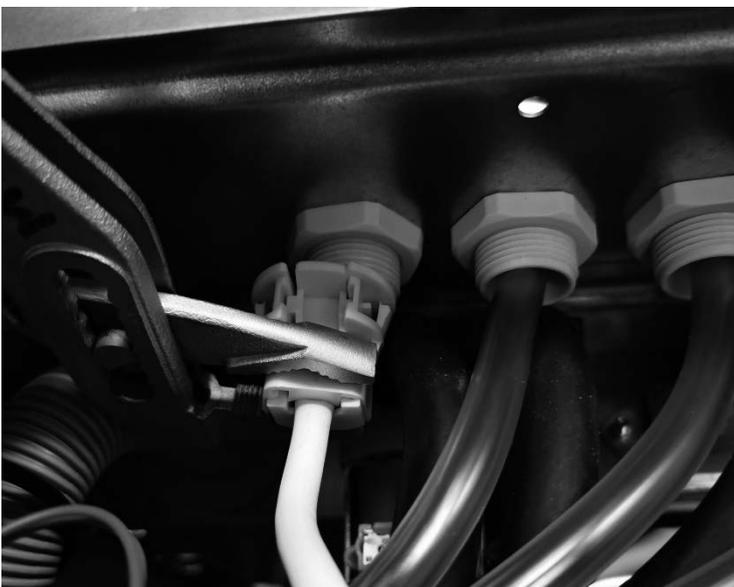
12. Use strain relief that was in the kit, mount it to the cable from inner side of washing machine right next to grommet, make sure no gap is left between grommet and strain relief. Squeeze strain relief tight with appropriate tool (pliers).
