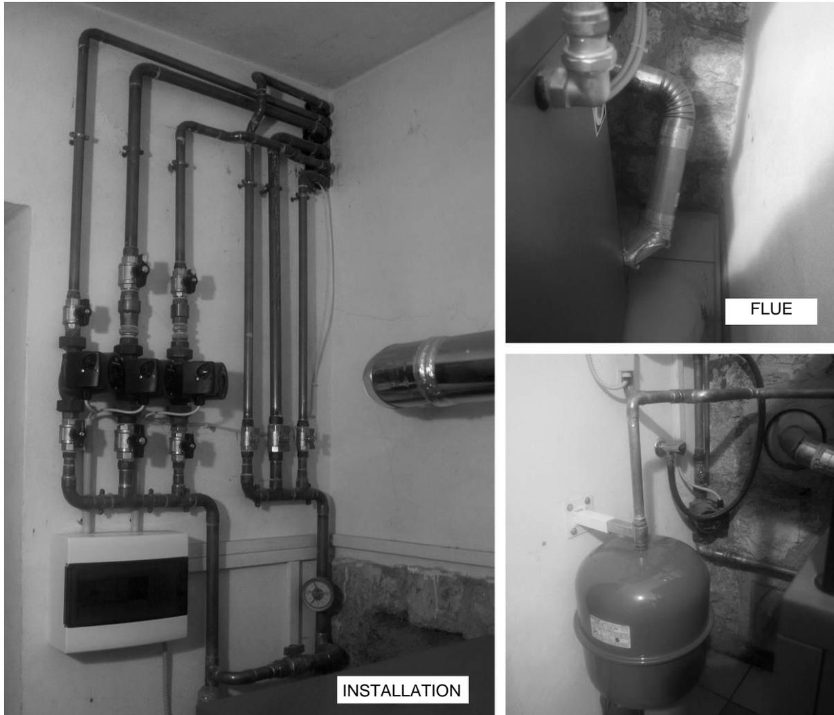
*Figure 14: Boiler room example*
